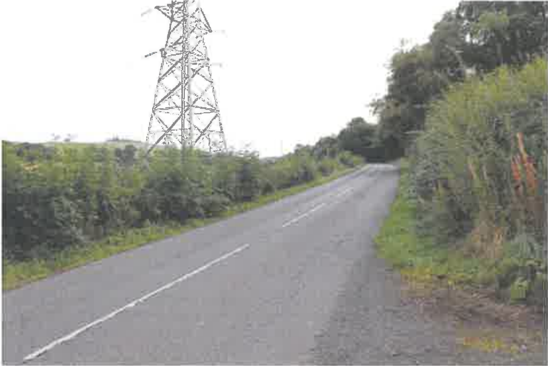
To Rink Hill from A707 electric substation entrance
